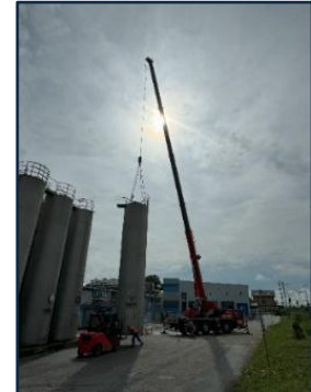
Fig.2 Dismantling of a raw material silo at the old site
