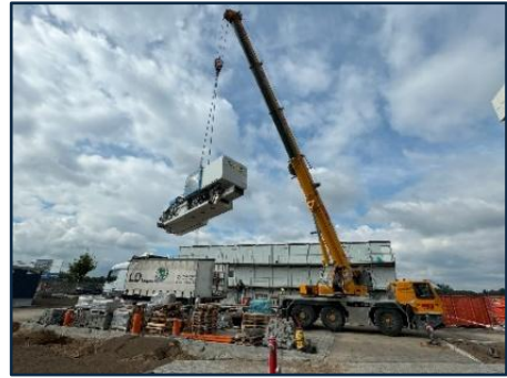
Fig.18 The loading of a production machine at the old site in Bensheim
