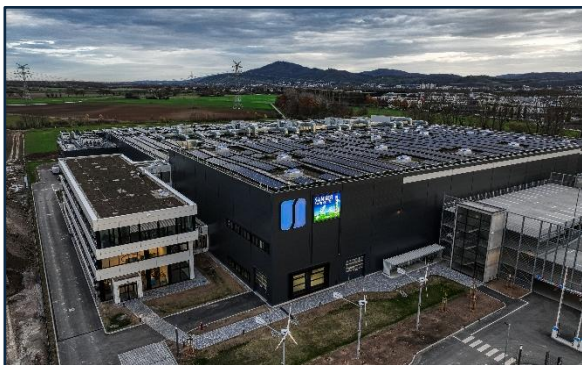
Fig.4 The PV system at the new site at Bensheim
